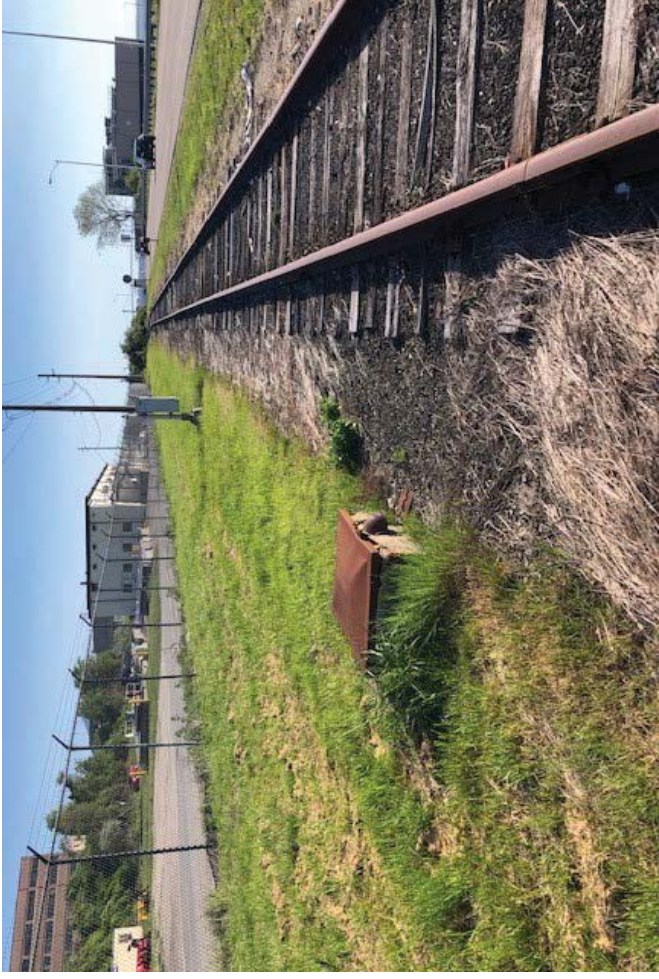
38. Typical concrete box, Middletown.
