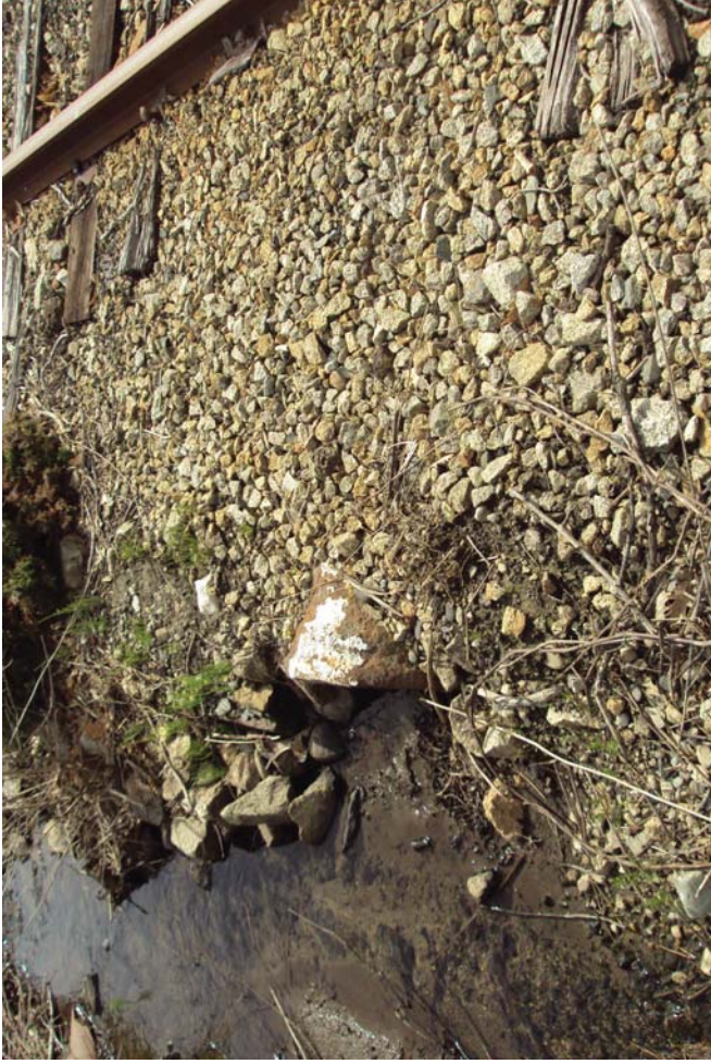
29. Typical cast-iron culvert, Portsmouth.
