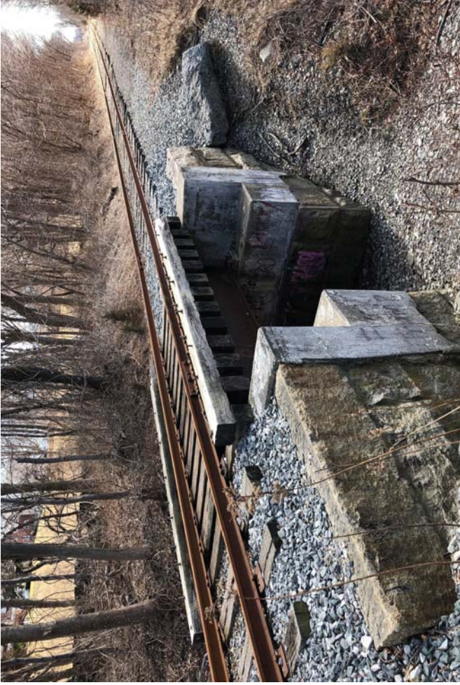
21. Bridge over dry bed, deck-plate girder with granite block and concrete abutments, Portsmouth.
