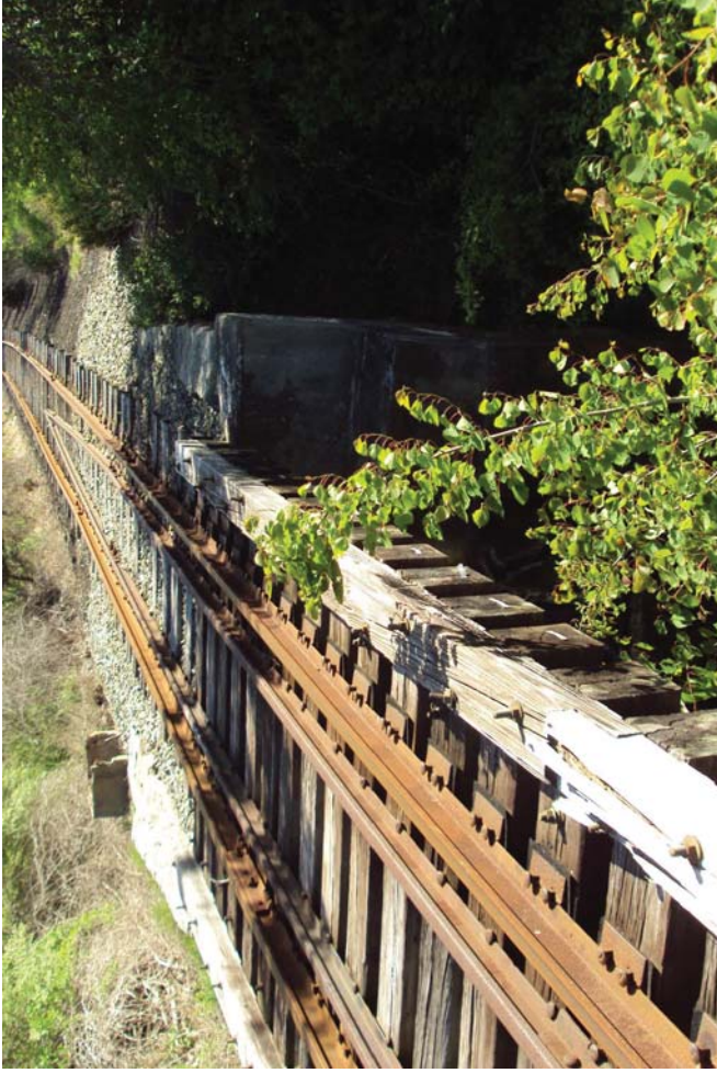
33. Bridge over private drive, deck-plate girder with granite block and concrete abutments over former private drive, Middletown.
