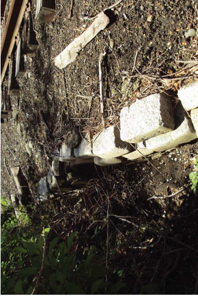
41. Cast iron culvert with modern granite block abutment, Middletown.
