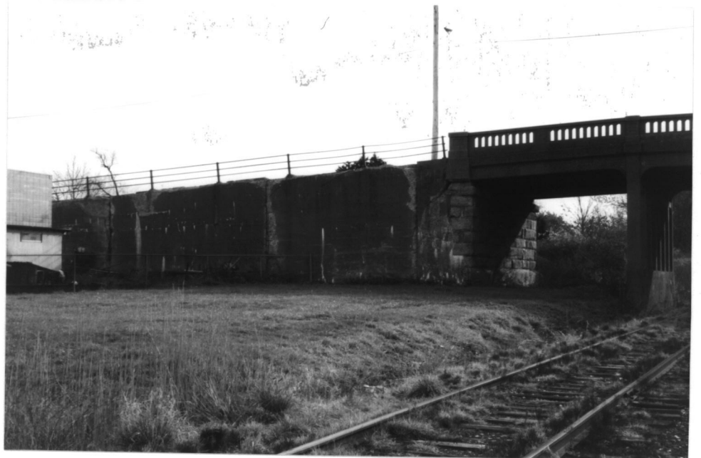
View north side elevation: west abutments and approach span NP(94) PAL(579)-2-21
