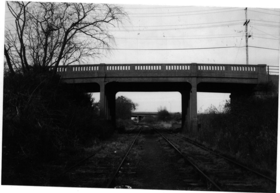
Side elevation View south NP(94) PAL(579)-2-16
