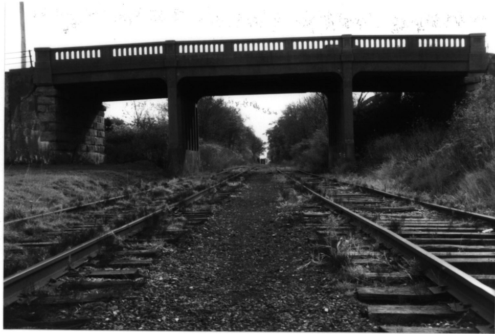
View north side elevation: NP(94) PAL(579)-2-20
