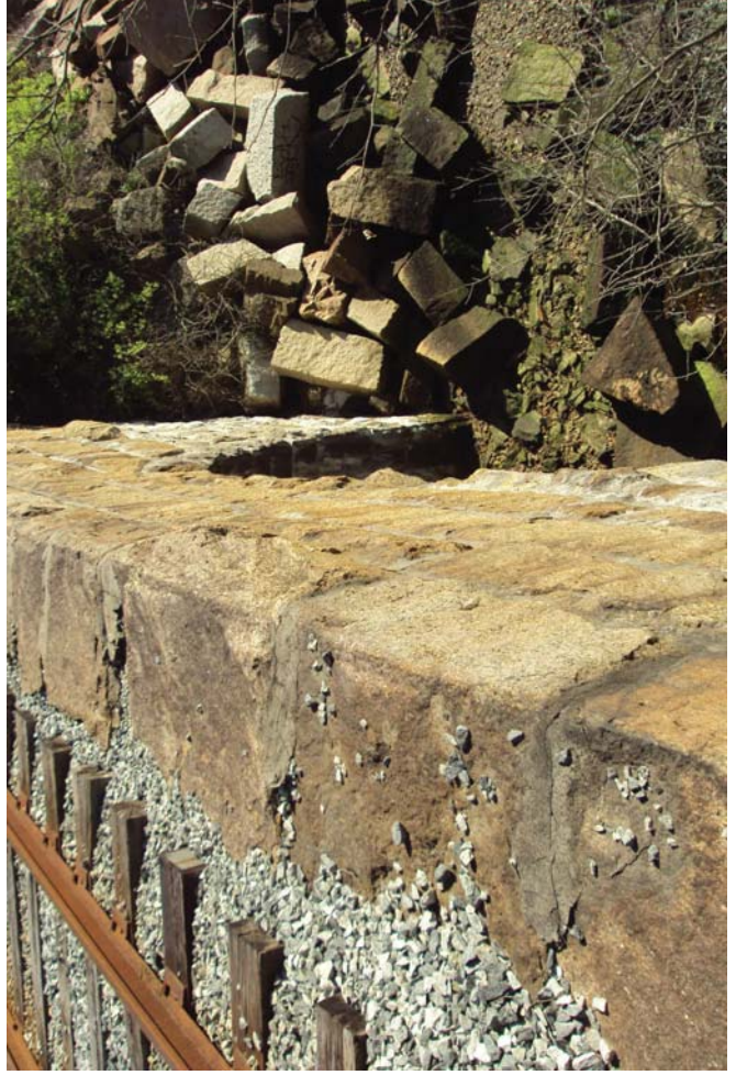
35. Bridge over unnamed brook, Stone arch, granite block bridge over unnamed Brook south of Greene Lane, Middletown.
