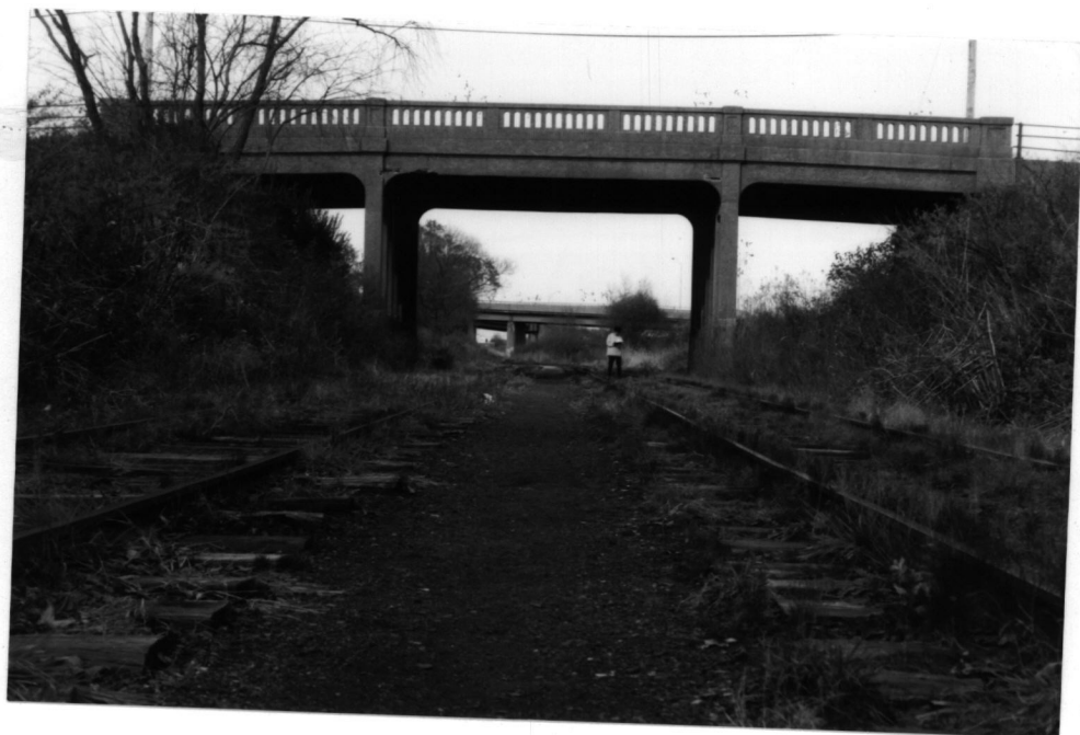
Side elevation View south NP(94) PAL(579)-2-17
