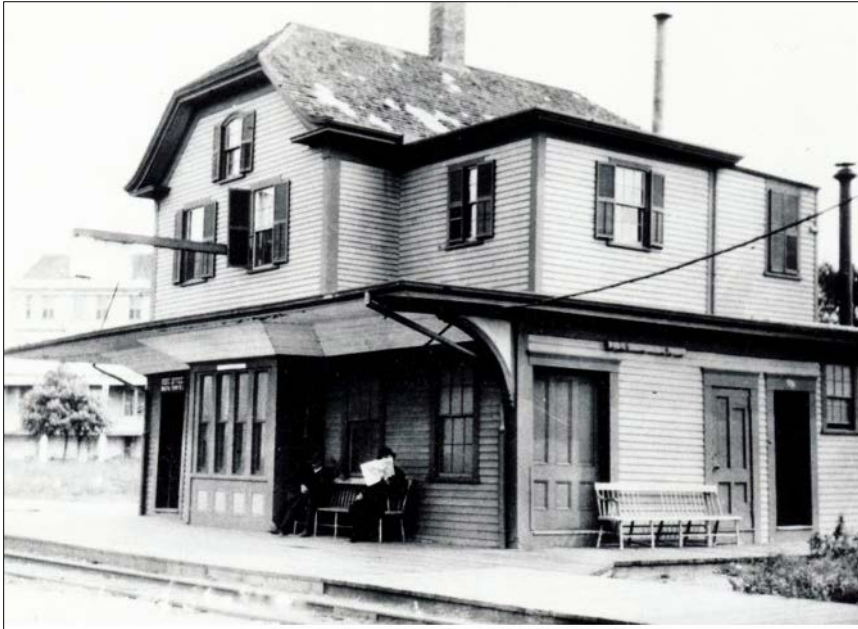
Figure 5. Bristol Ferry Station, Portsmouth n.d. (source: Ozog 2019).
