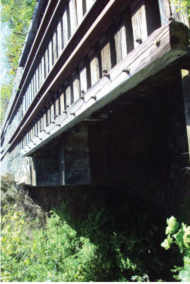
34. Bridge at terminus Greene Lane, deck-plate girder with granite block and concrete abutments, Middletown.
